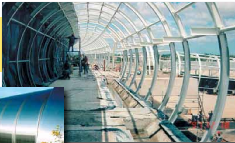
Fortaleza Airport Fortaleza, Brazil, 1998 Stainless steel panels bonded to steel frame.
