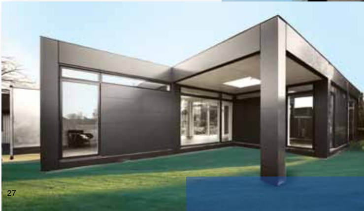
Private Residence by Qbes Skanderborg, Denmark, 2007 Facade bonding 3M VHB Tape W20F
