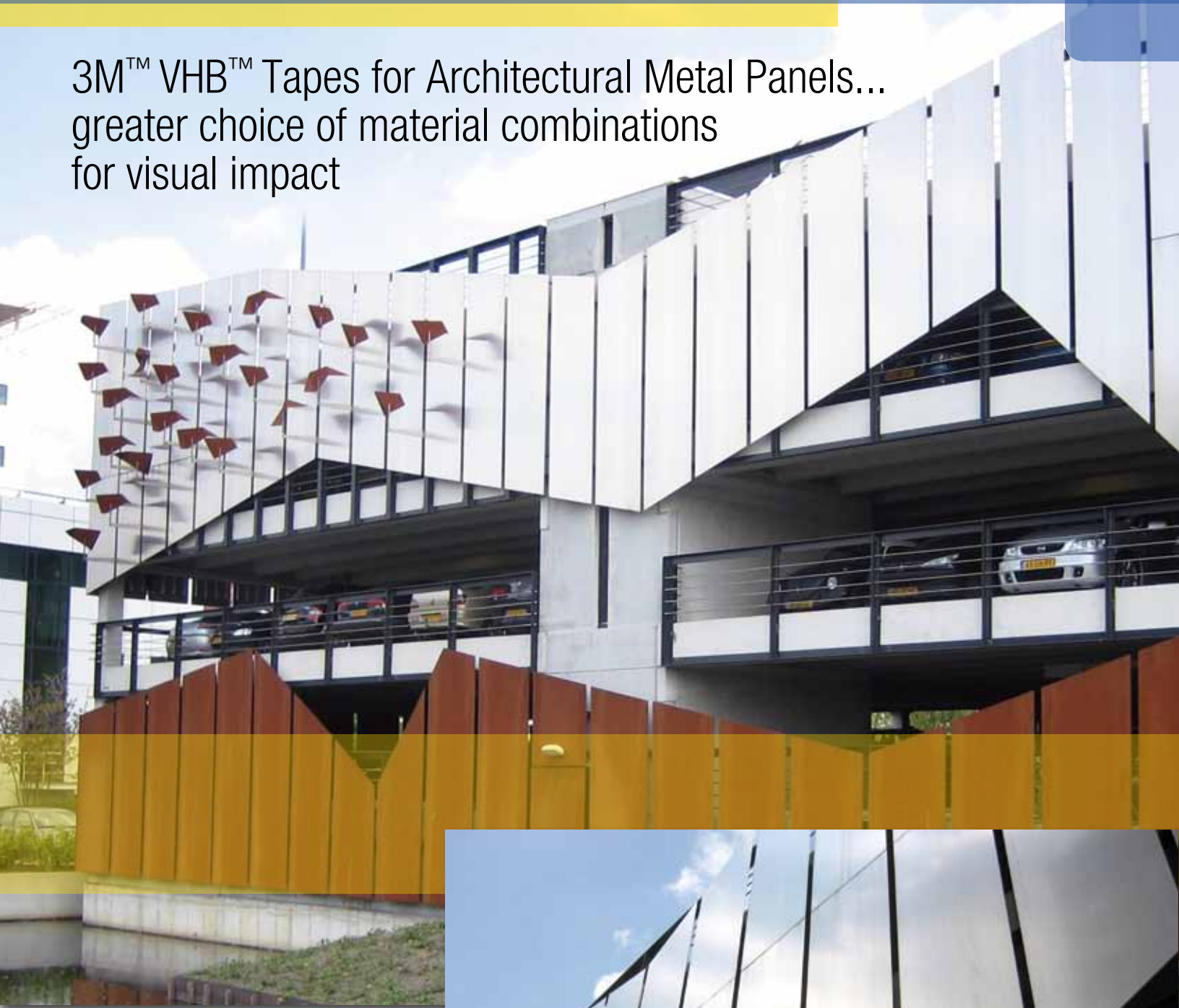
Pettlaarspark Den Bosch, Netherlands, 2006 Fabricator: Sorba Aluminum panel bonding 3M™ VHB™ Tape W20F
