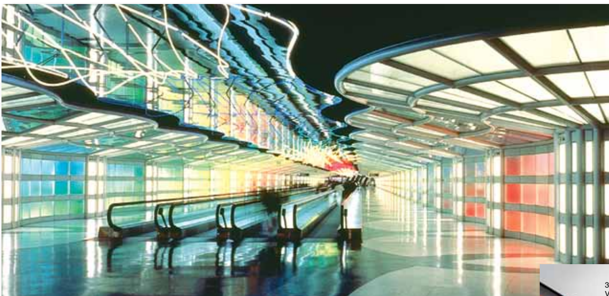
O'Hare Airport, Chicago, IL, USA Architect: Custom Products of Southgate, CA, 1987 Mirror-finish composite ceiling panels bonded to a suspension frame.
