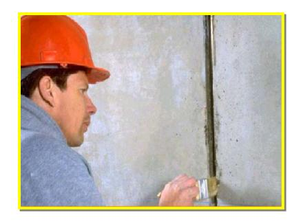
Proper primer application with brush ponding, waiting time Prime only sides of the joint. Primer outside the joint may stain the substrate. Prime & seal the same day
