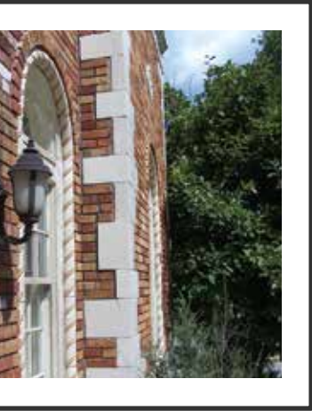
Re-anchoring to metal stud with Stitch-Ties
