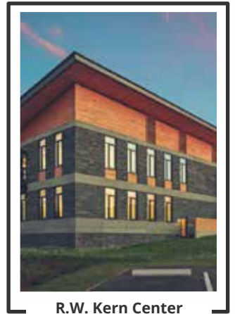
R.W. Kern Center at Hampshire College
