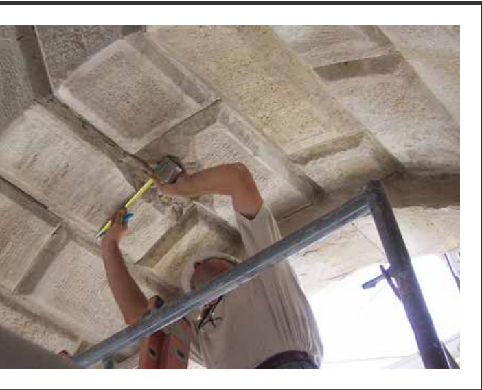
Re-anchoring terra cotta with Stitch-Ties
