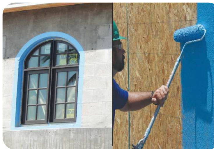
INSTALLATION NOTE: Field application should be completed prior to setting the Window/ Door package.
