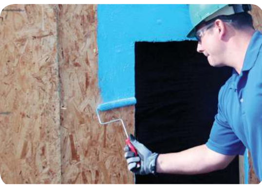
INSTALLATION NOTE: Be sure to use a 4- or 6-inch, hot-dog-style roller handle and mini roller with a high density foam cover that will give you the best yields and coverage.
