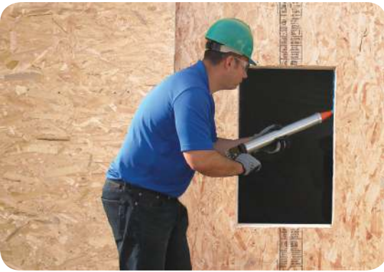
INSTALLATION NOTE: All openings and voids are to be filled flush with Blue Barrier Joint Filler 2200.
