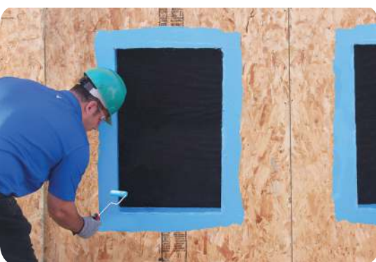
INSTALLATION NOTE: Be sure to use a 4- or 6-inch, hot-dog-style roller handle and mini roller with a high density foam cover that will give you the best yields and coverage.
